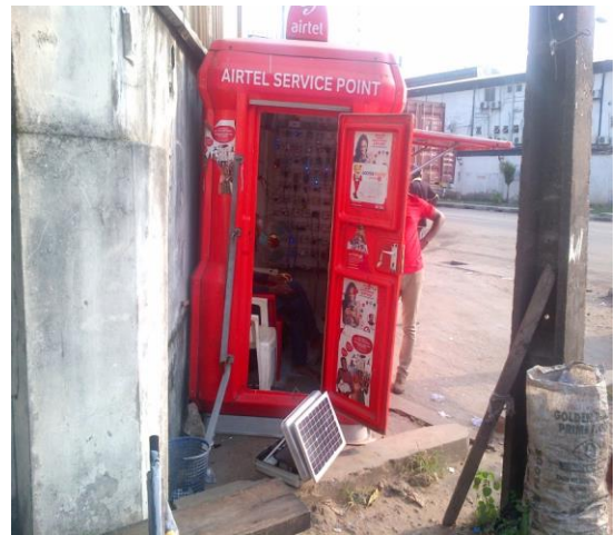
Fig. 9: PCB powers service point sockets
